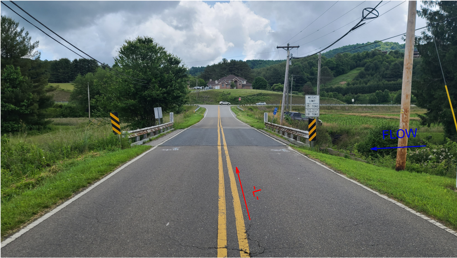
VIEW FROM WEST OF EXISTING BRIDGE LOOKING EAST ALONG SR 1100
