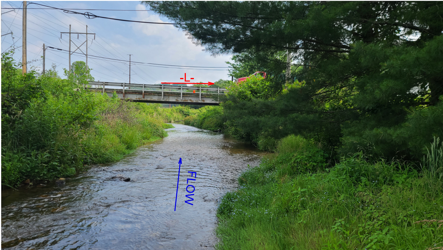
VIEW FROM SOUTH OF EXISTING BRIDGE LOOKING NORTH
